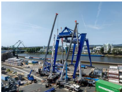
Photo 5: Relocating the cranes to ensure maximum efficiency.
